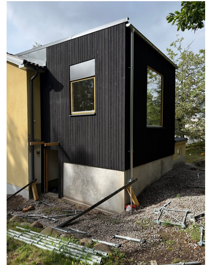
New extension (under construction)
