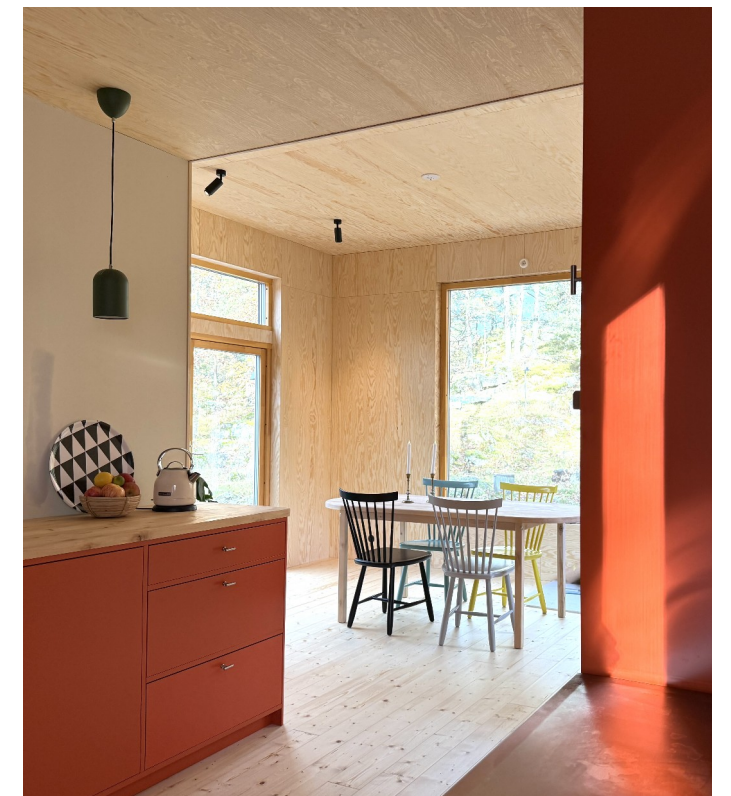
New kitchen (under construction)
