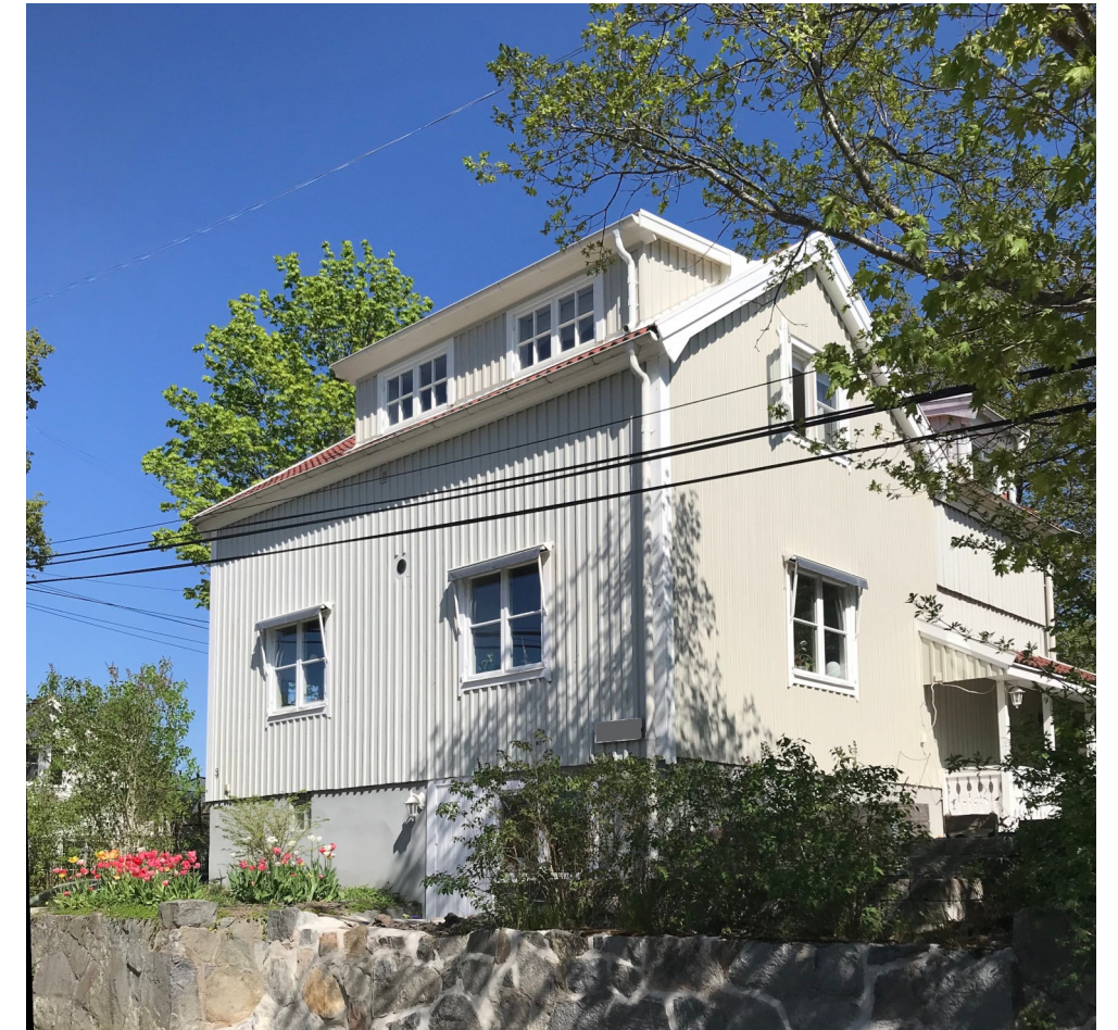
Street facing facade. Visible are the new dormer window and the reconstruction of an existing external staircase / retaining walls.
